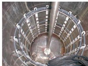
Figure 1: Multiple electrodes fitted to a stir tank
